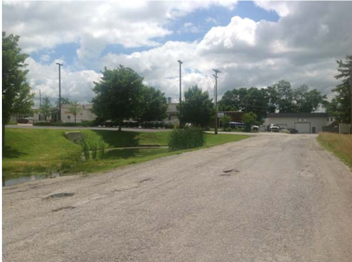
Wet area and possible subgrade problems on connector road near Early Learning Village.
